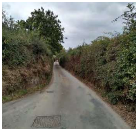
Left: Narrow steep lanes with banked hedges channel runoff rapidly downhill.
